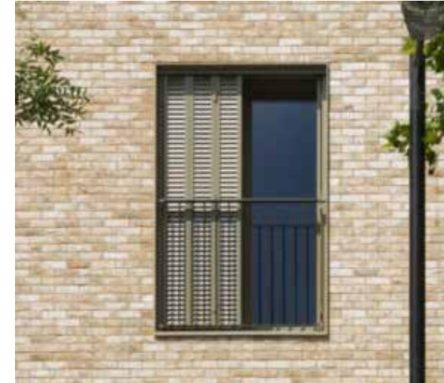
Window with integrated ventilation screen. Future Homes, Passivhaus, Southwark Maccleanor Lavington
