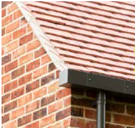
Mortared roof verge
