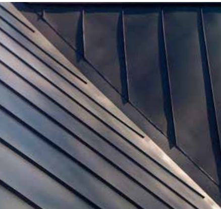
Folded standing seam roof and walls
